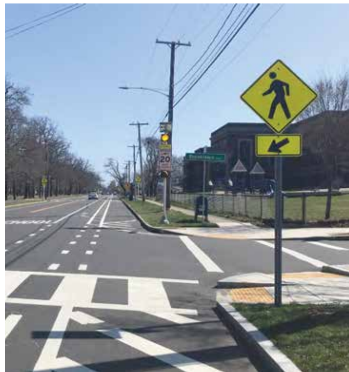
Safe Routes to School project at Ashley and Lincoln Elementary Schools in New Bedford created curb bump-outs, ADA-compliant accessible ramps, bike lanes, and replaced school zone flashers.
